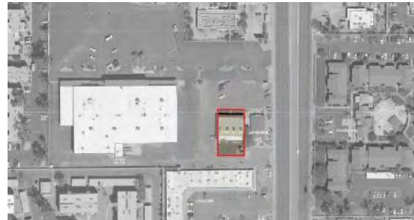
Parcel does not have adequate space for parking, and does not have access to a public roadway
